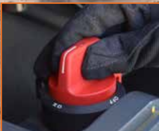
Battery cut-off switch
